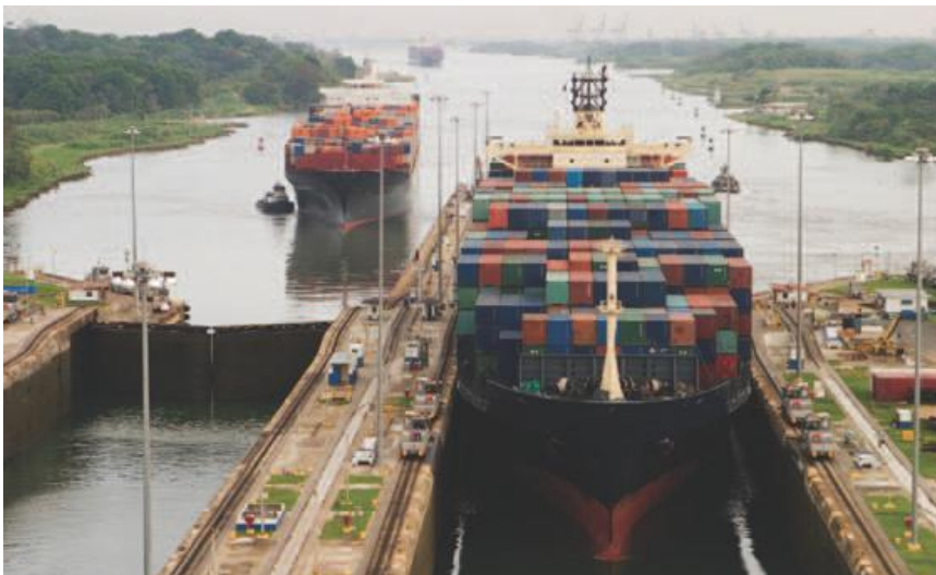
Ship passing through a Panama Canal Lock.
