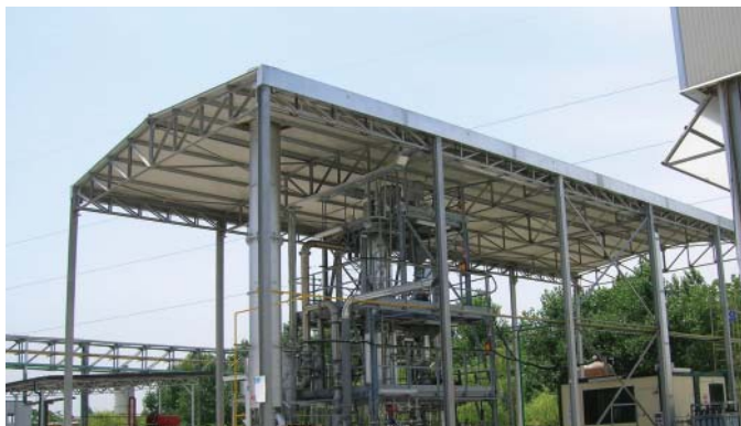
Fig. 2: AMRA FluGas Pilot Plant
